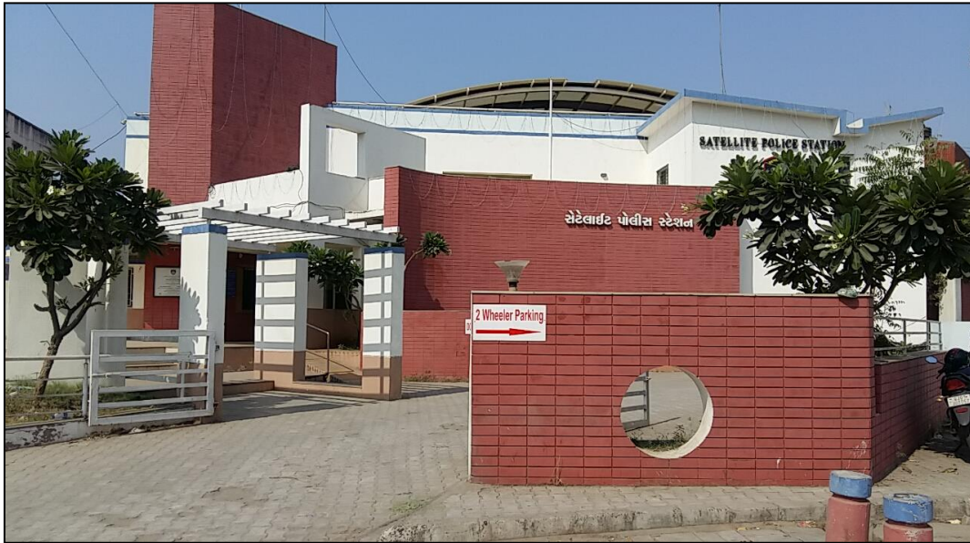
Image:- Satellite Police Station, Ahmedabad, Gujarat
